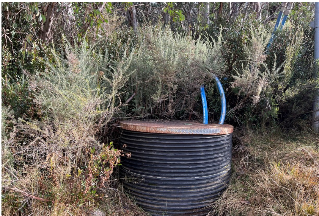
Figure 3: Example of Steel Pit for Lance Guns
